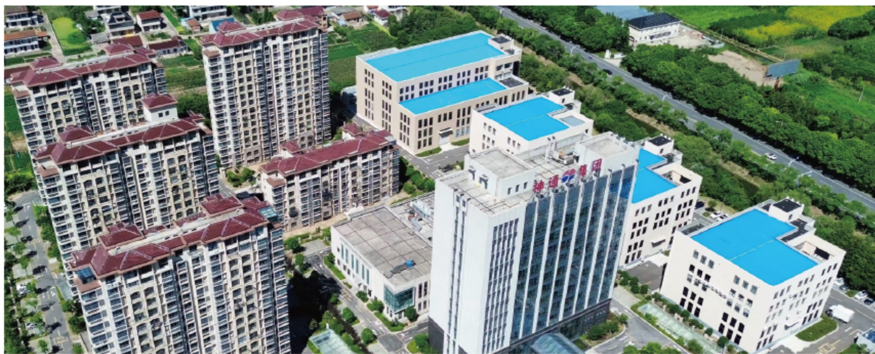
STV HEADOFFICE & New energy valve base Pipe/Valve for Hydrogen, Military and special scenes Land area: 34,167.5 m²
